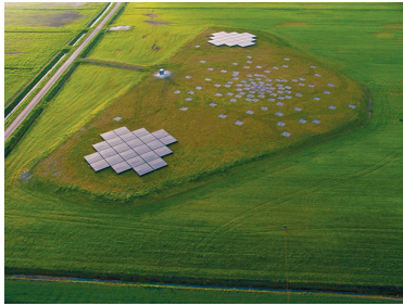
LOFAR Station in Drenthe NL
