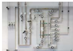
Gas bottle and distribution Cabinets
