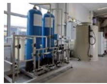
Chemical distribution DI Water system
