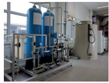
Chemical distribution DI Water system
